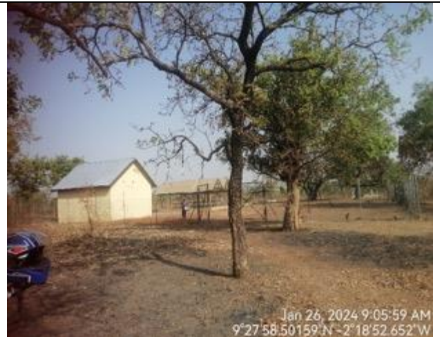
Soma processing plant
