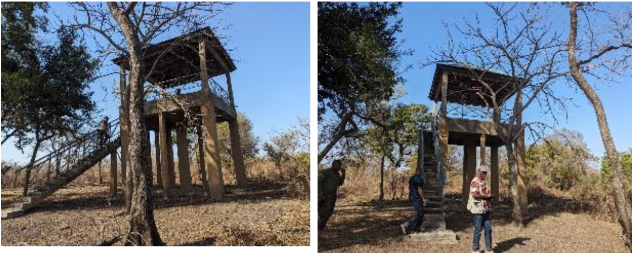
Figure 3-2: Existing Game Viewing Platform at Gbele Resource Reserve
